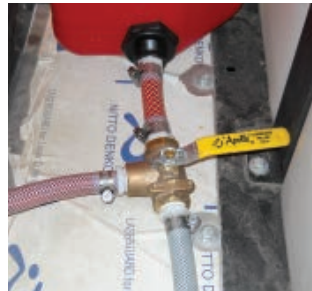
Valve position for antifreeze
